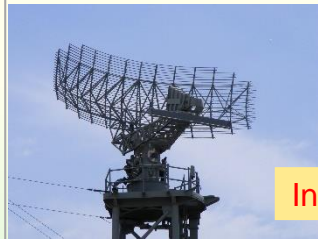
Aerodrome Surveillance Radar
